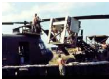
Blade Change with forklift
